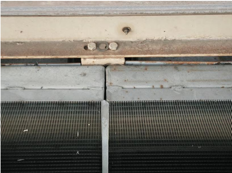
Joint with caulking – Red Bluff flat plate screen (screens bolted to supports).
